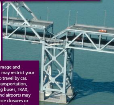
The 1989 magnitude 6.9 Loma Prieta earthquake caused this section of the San Francisco-Oakland Bay Bridge to collapse. (Photo courtesy of USGS)
