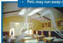
Failure of fluorescent light fixtures in the Dawson Elementary School Library during the 1983 Coalinga, California, earthquake. (Earthquake Engineering Research Institute photo)
