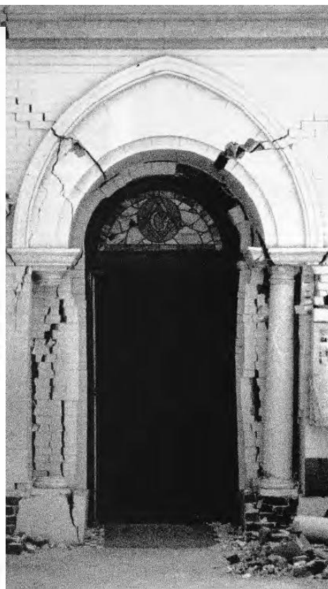
Figure 3.2: The impact of building configuration on seismic performance has only begun to be recognized in building codes. A wide range of existing buildings have been designed without taking such considerations into account, such as this soft first story example in San Francisco.
