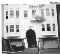
Figure 3.2: The impact of building configuration on seismic performance has only begun to be recognized in building codes. A wide range of existing buildings have been designed without taking such considerations into account, such as this soft first story example in San Francisco.
